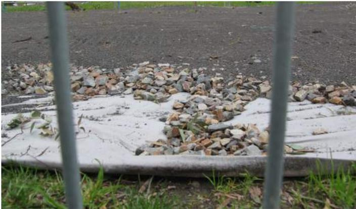
Figure 2: Geotextile fabric laid between natural ground and the road base reduces the amount of road base required, and the underlying soil profile is not disturbed or contaminated
