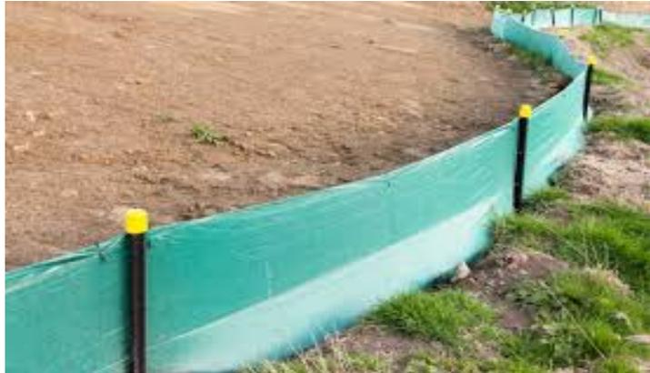
Figure 4: Woven sediment fence at lowest lying boundary to prevent sediment run-off from site.
