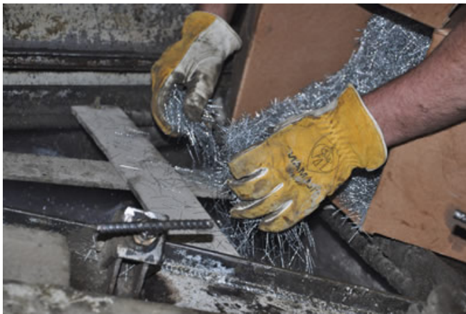
Figure 2: Adding Helix Micro Rebar to concrete mix
